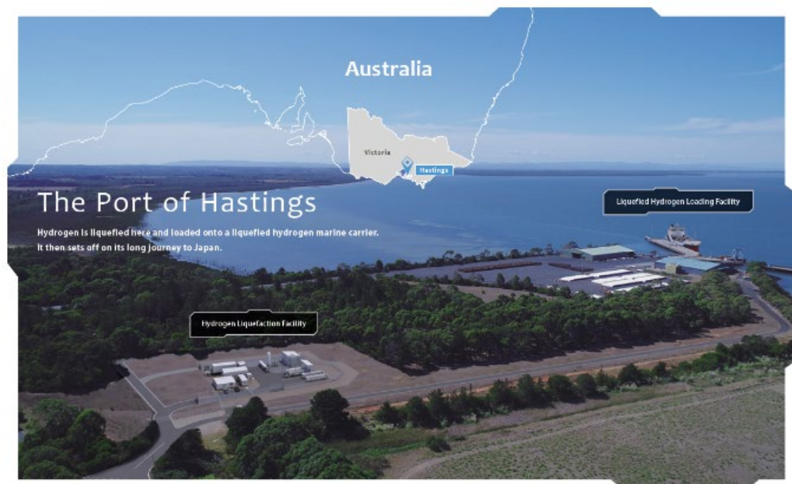
Figure 14 Port for liquid hydrogen in Hastings, Australia [HYSTRA-Project]
