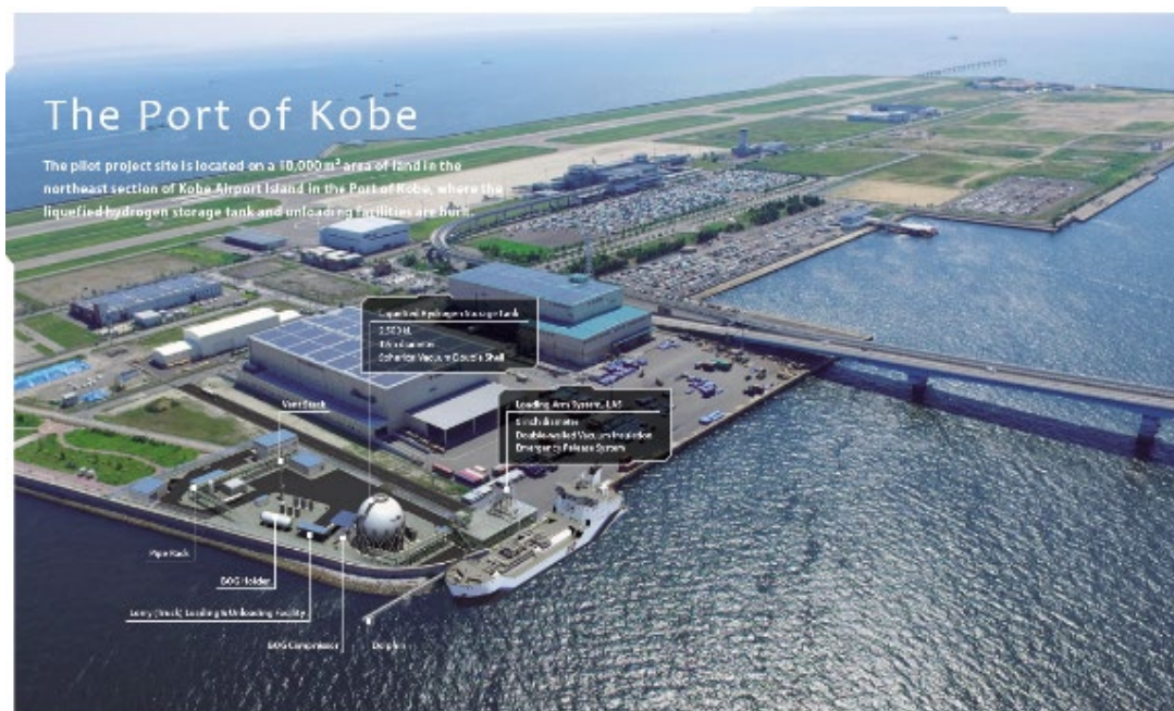
Figure 13 Port for liquid hydrogen in Kobe, Japan [HYSTRA-Project]
